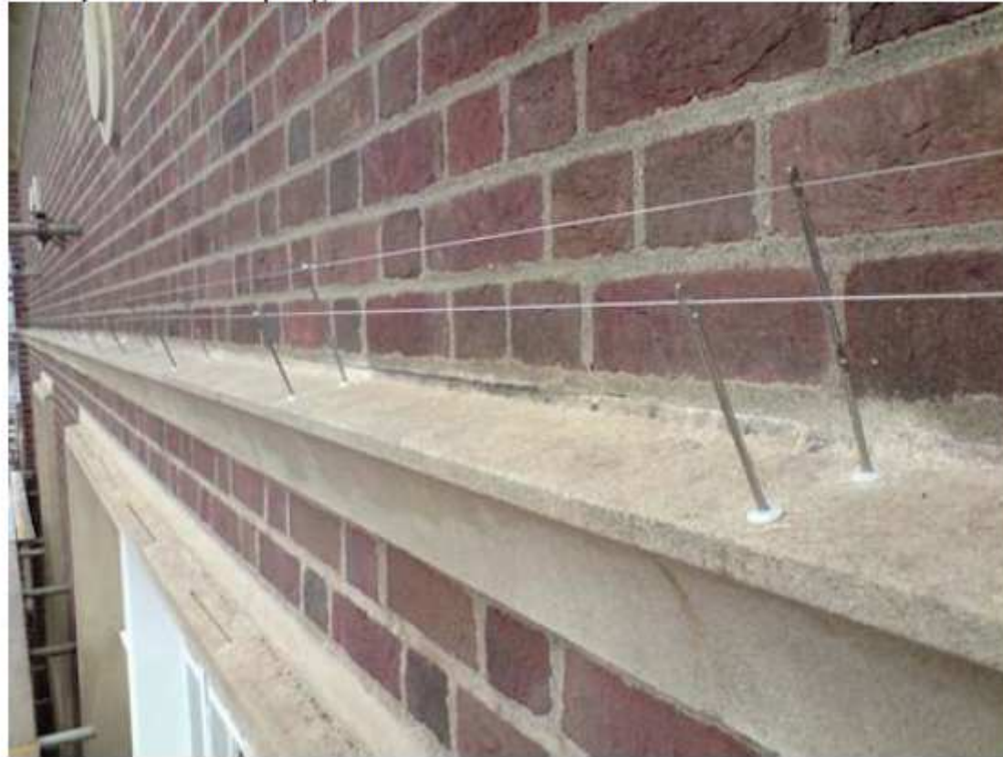
Example of 2 rows spring wire.
